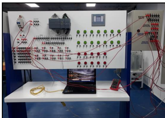
Fig. 1. Tablero de control PLC
